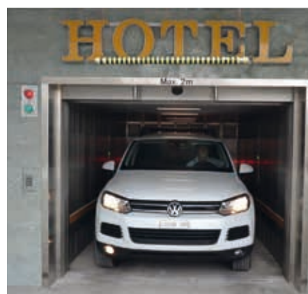
Garage Swissotel - Zürich, Switzerland
