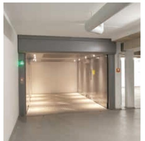
Rolling gate and traffic lights in a discreet appearance in the lower position.
