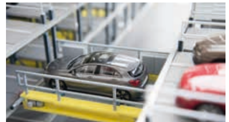
Under construction BLOX, COPENHAGEN, DENMARK Fully automated car park system with almost 320 parking spaces
